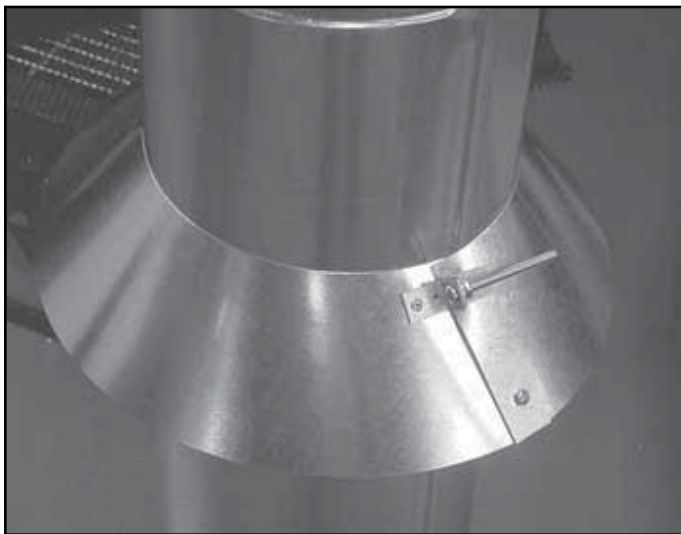
Figure 10.14 Assembling the Storm Collar Around the Pipe
